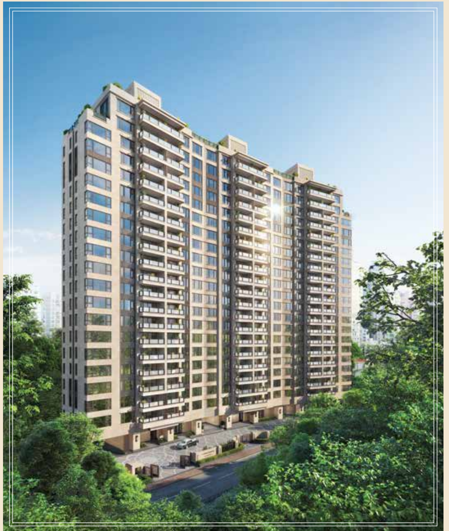
ST. GEORGE'S MANSIONS FAÇADE FACING KADOORIE AVENUE 1,2,3,5
