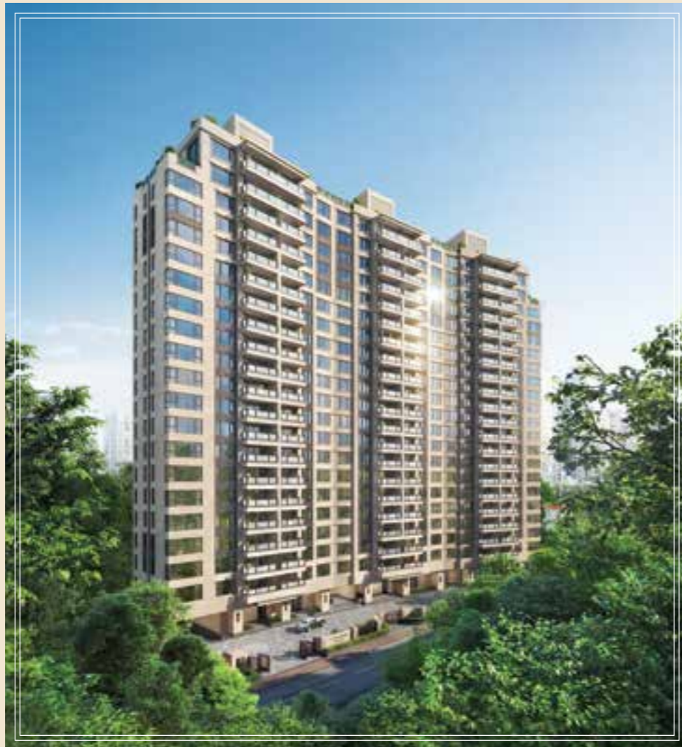
ST. GEORGE'S MANSIONS FAÇADE FACING KADOORIE AVENUE 1,2,3,5
